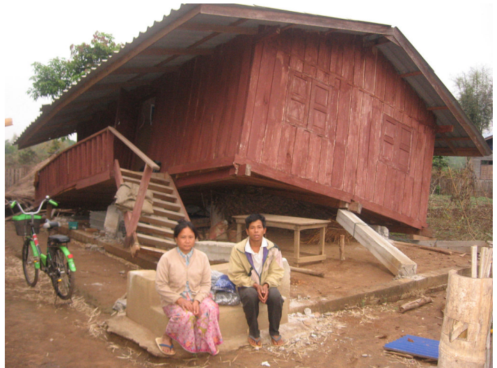
HOUSE OFF PIERS
